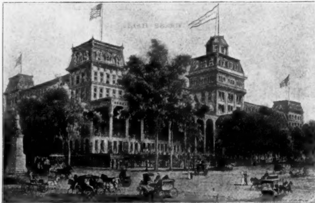
GRAND UNION HOTEL, BROADWAY FACADE.
